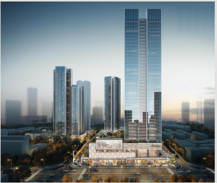
卓越珺奕府办公楼 EXCELLENT JUNYI MANSION OFFICE BUILDING
