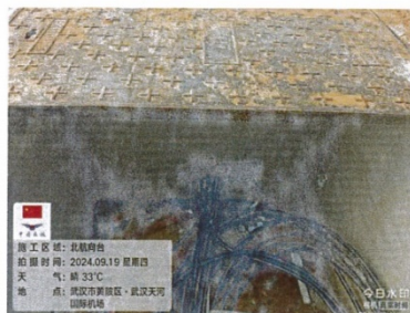
通信井进方舱管路封堵
